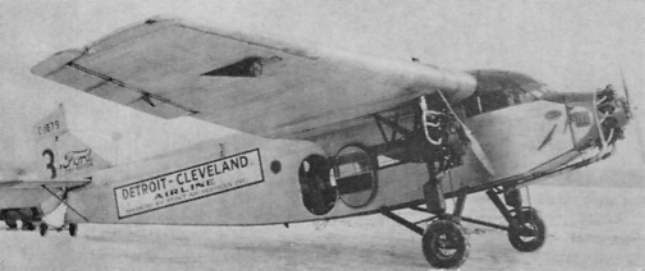
The 4-AT-A, first production model. This plane, the fifth built, shows the early design with engine exhaust going up through the wing. A 1927 photo showing early Stout Air Services.
