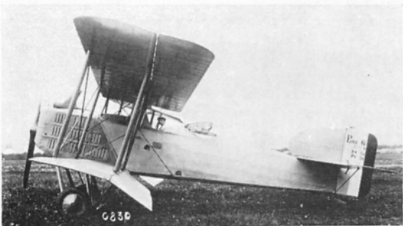
Two views of an early Breguet 14B2, No. 670. The three-quarter front view shows the greater length of the lower wing; both illustrations show the lower-wing flaps clearly. This aircraft had not been fitted with Michelin bomb racks and their characteristic forward projection of the lower-wing leading edges when this photograph was made; there were no windows in the fuselage sides at the observer's cockpit, and his gun ring was a T.O.4. No shutters were fitted to the radiator at this stage.
