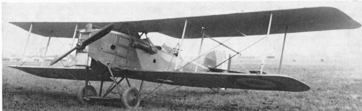
Fiat-powered Breguet 14A2 with enlarged radiator.
