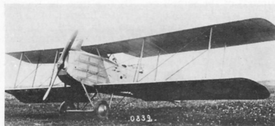
Two views of an early Breguet 14B2, No. 670. The three-quarter front view shows the greater length of the lower wing; both illustrations show the lower-wing flaps clearly. This aircraft had not been fitted with Michelin bomb racks and their characteristic forward projection of the lower-wing leading edges when this photograph was made; there were no windows in the fuselage sides at the observer's cockpit, and his gun ring was a T.O.4. No shutters were fitted to the radiator at this stage.
